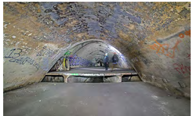
Ouseburn sewer. Photo Chris Rayner
